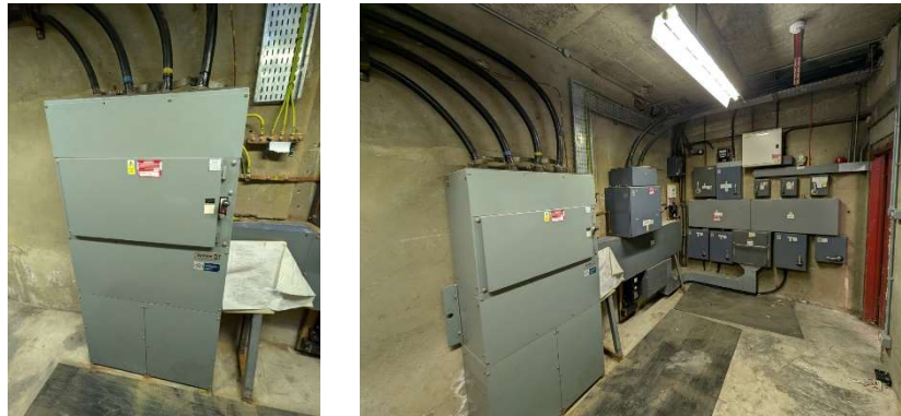
Photos: Intake Cubicle and Main Busbar Chamber
