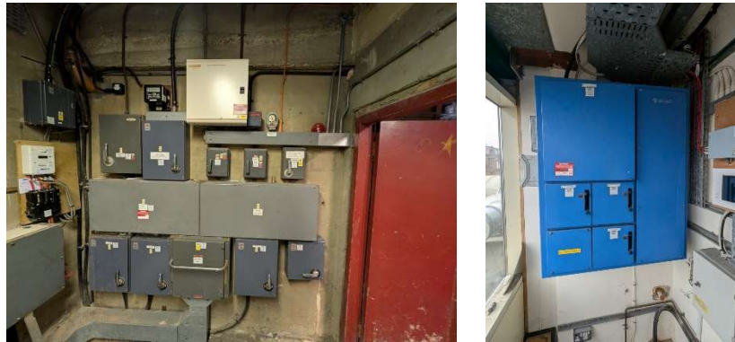
Photos: Landlord's Busbar Chamber, Fuse Switches and Distribution Boards
