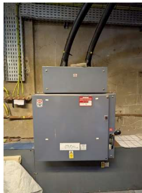
Photos: Tenant's Main Isolator and Sub-Main Cables
