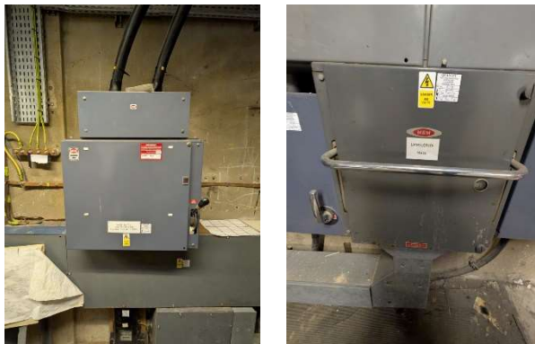
Photos: Tenant's and Landlord's Fuse Switch Isolators
