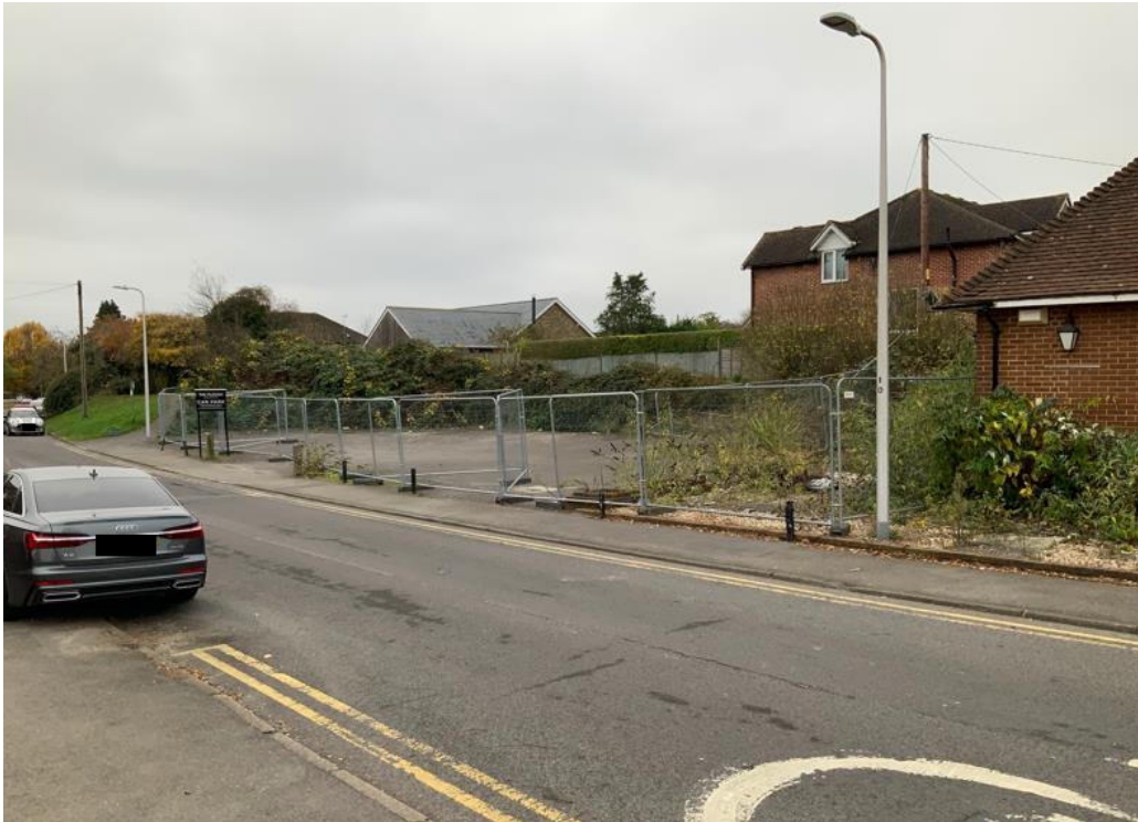
Photograph 5: View looking south west across site showing vegetation encroachment
