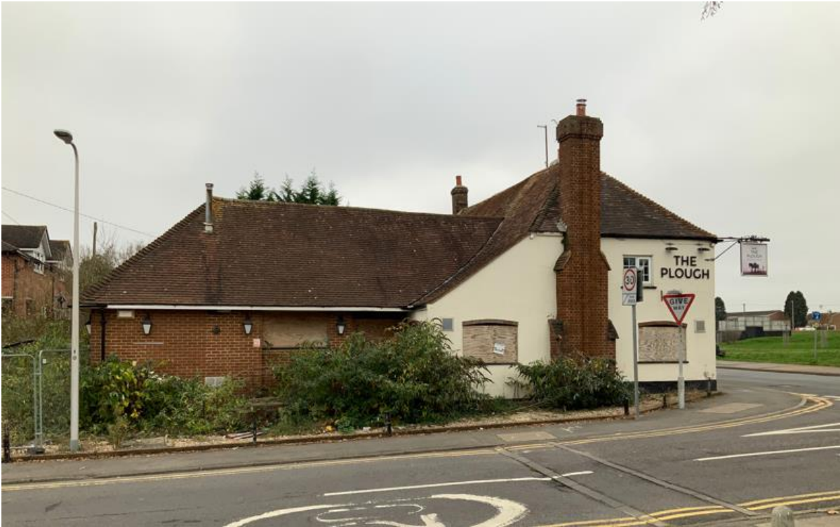
Photograph 3: View of the former public house from across Stoney Lane
