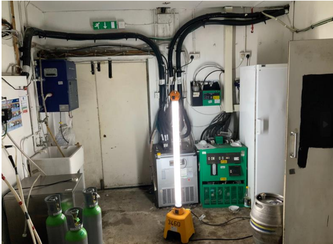
Photograph 7: Internal view of former alcohol room
