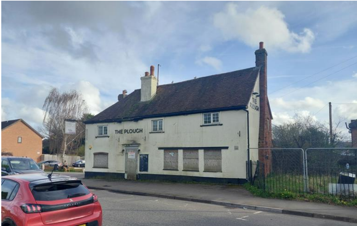
Photograph 1: View of the site from across Chapel Street
