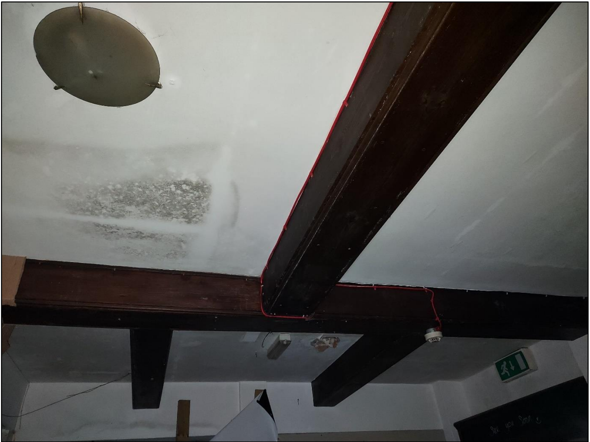
Photo 5: Boxed beams, later public house interior fittings
