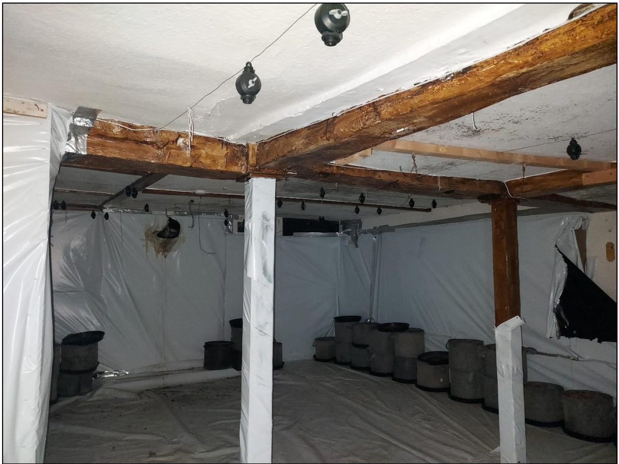
Photo 4: Internal historic timber beams and uprights
