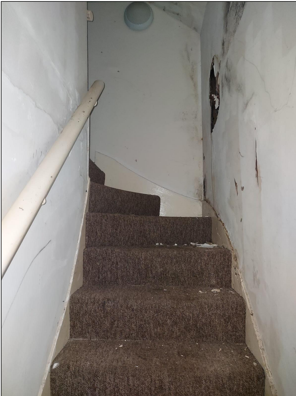
Photo 7: Carpeted timber stair to first floor
