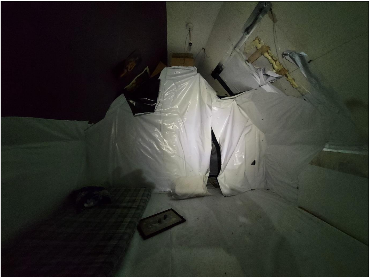
Photo 12: Upper part of rear extension
