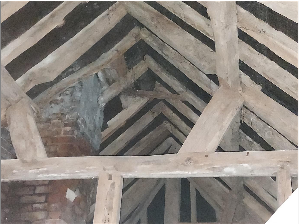
Photo 9: Historic, timber Queen post truss roof structure
