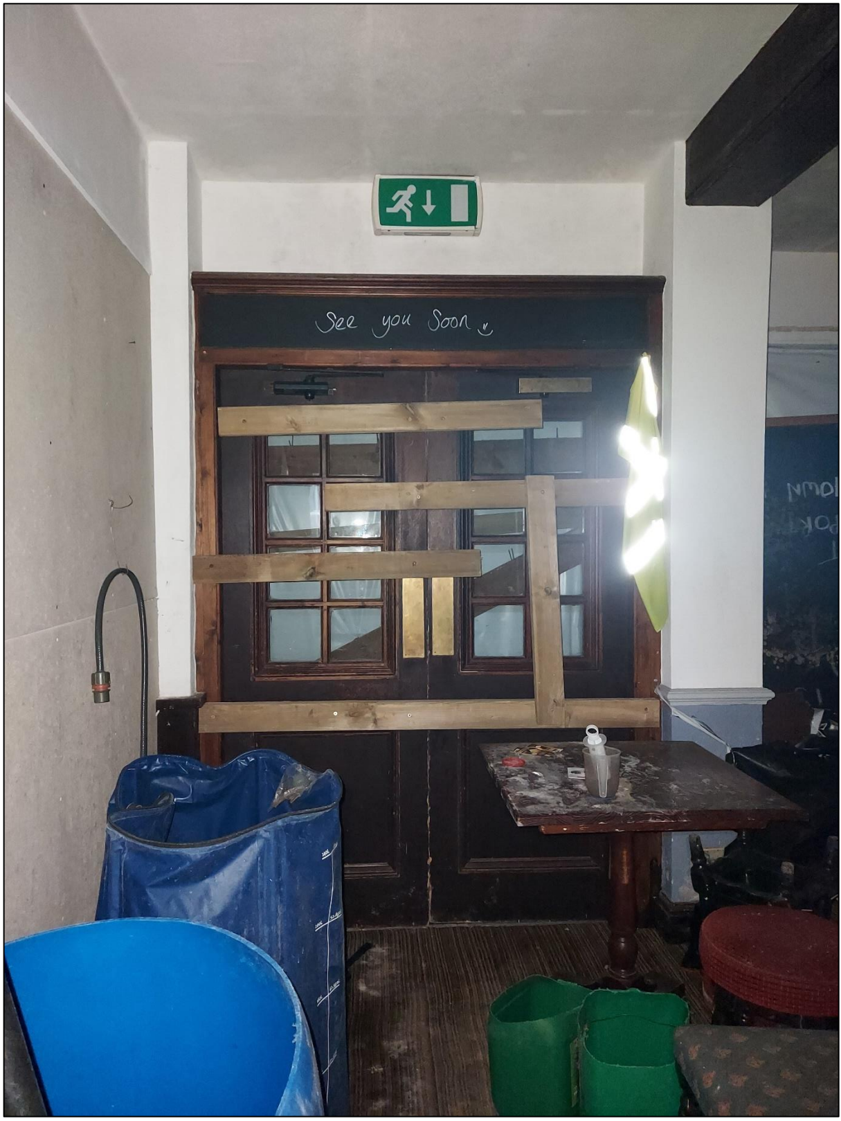
Photo 11: Ground floor, modern rear area
