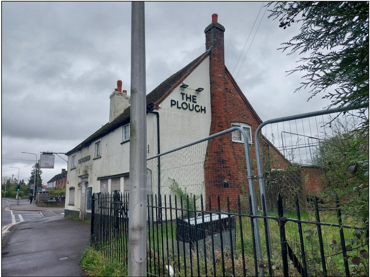
Photo 1: Northern and western elevation
