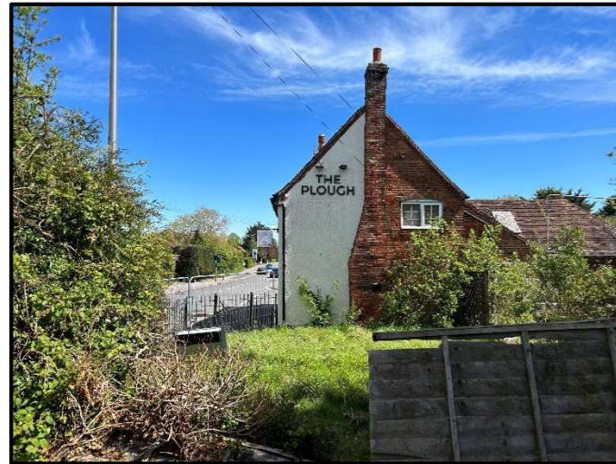
Photograph 1 View of the existing western elevation of The Plough Public House
