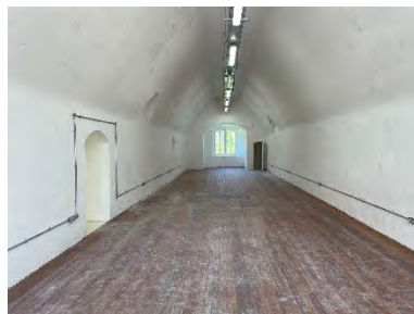
Plant Room (The Casemates)
