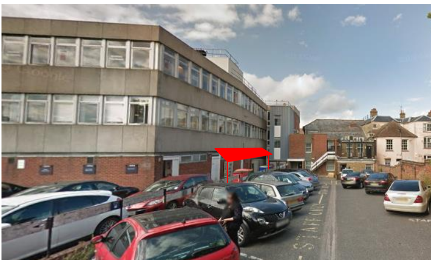
Figure 6.1 – Acoustic Screen/ Barrier.
